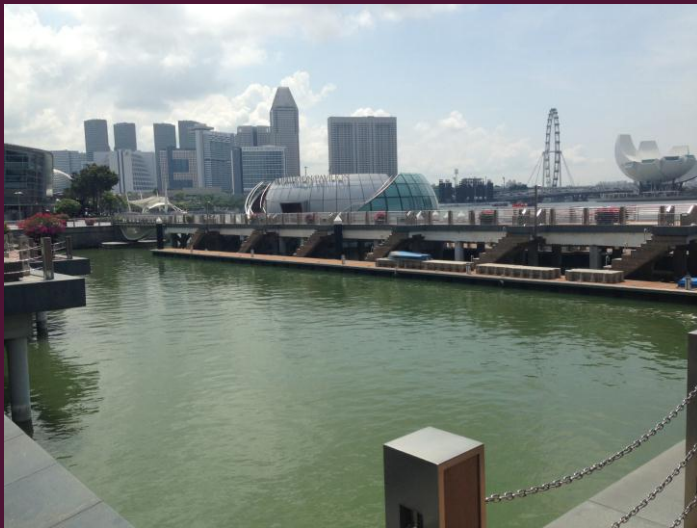
FINGER PIER JETTY
