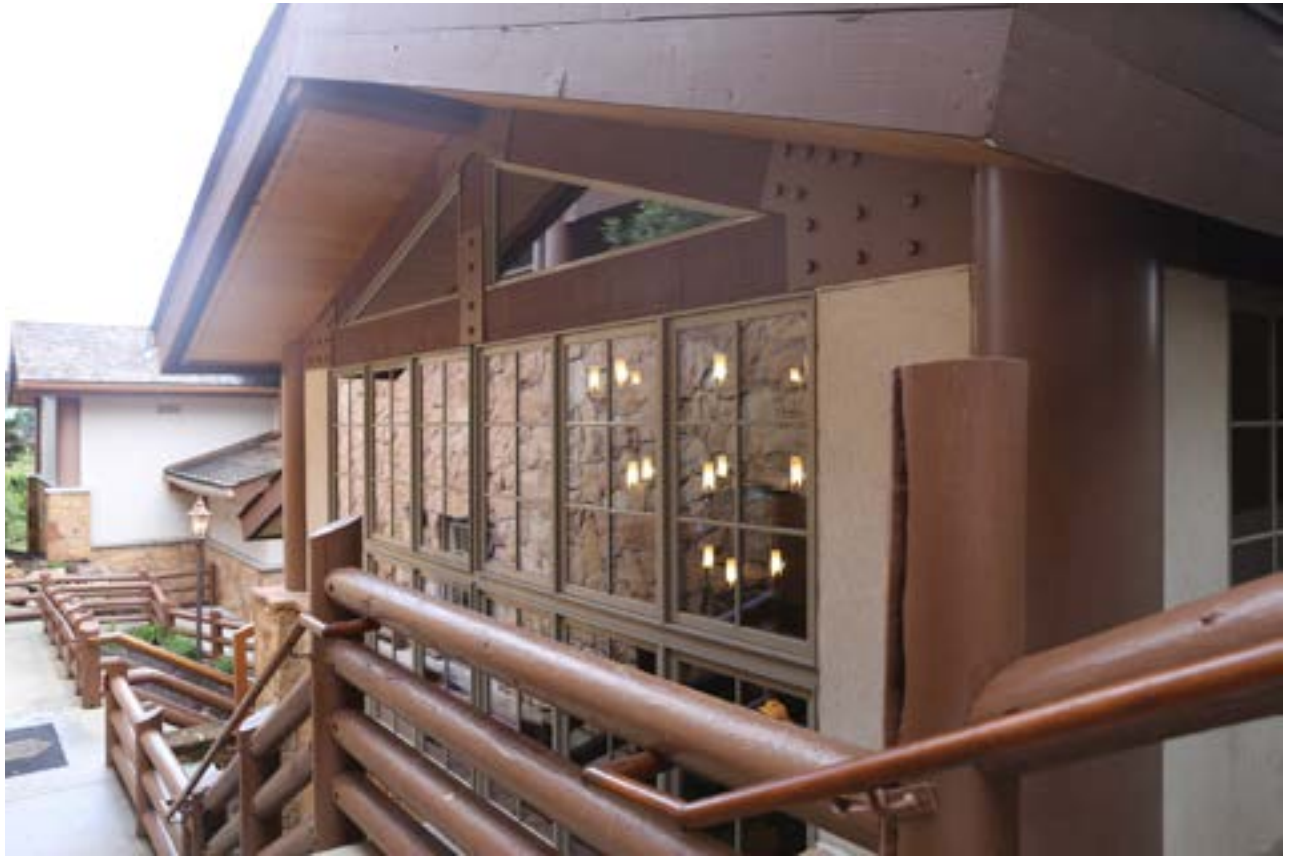
New spa and pool completed in 2001
