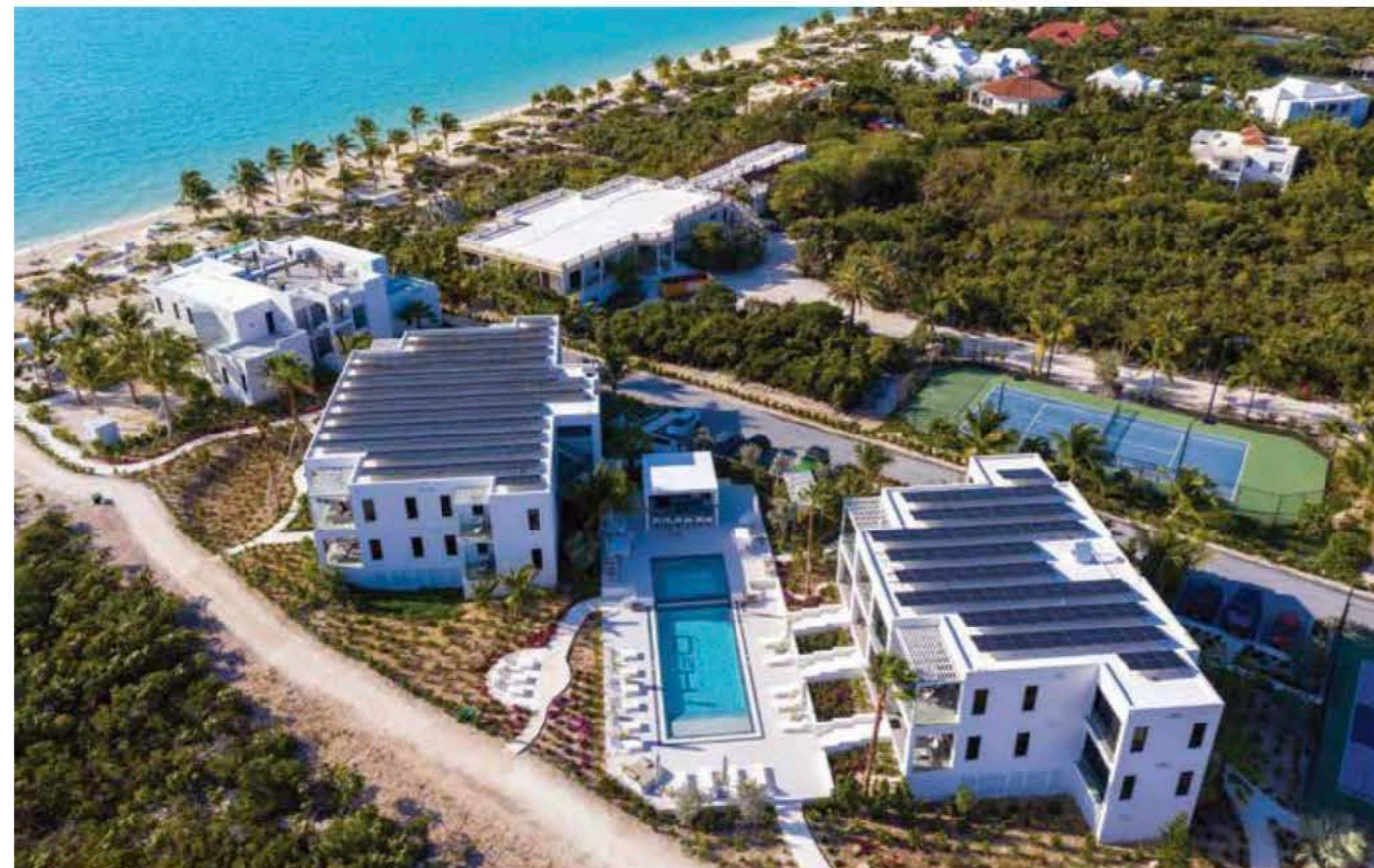
H2O Life. Style Resort includes three buildings on three acres of land fronting Long Bay Beach. Note the solar panels on the roofs. They contribute at least 1/2 of the electricity used by the resort.
