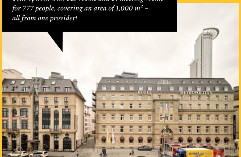
ONE-UNIT Flemings Hotel Frankfurt-Central & Metropolitan Hotel By Flemings
