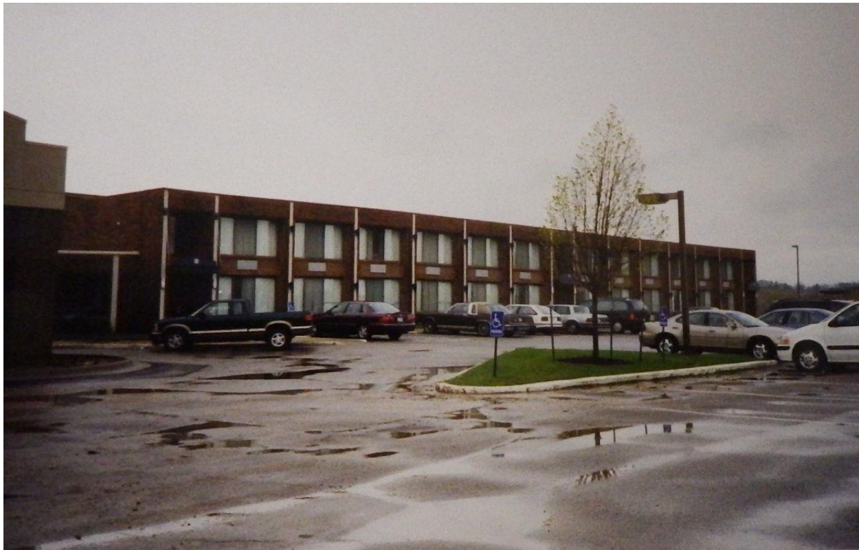
Figure 8-120: Radisson remodeling, south wall of south wing, 1997, looking northeast (Courtesy of Sheila Boyd)
