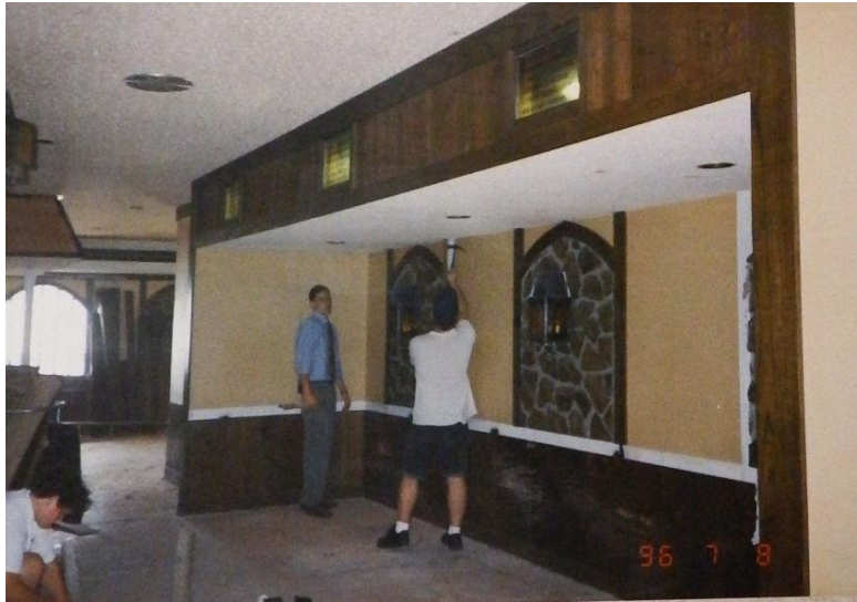
Figure 8-111: Former Royal Scot Dining room, note faux mansard, pointed arch windows with stone infill, stained glass, wainscot, 1996, looking south (owner scrapbook)
