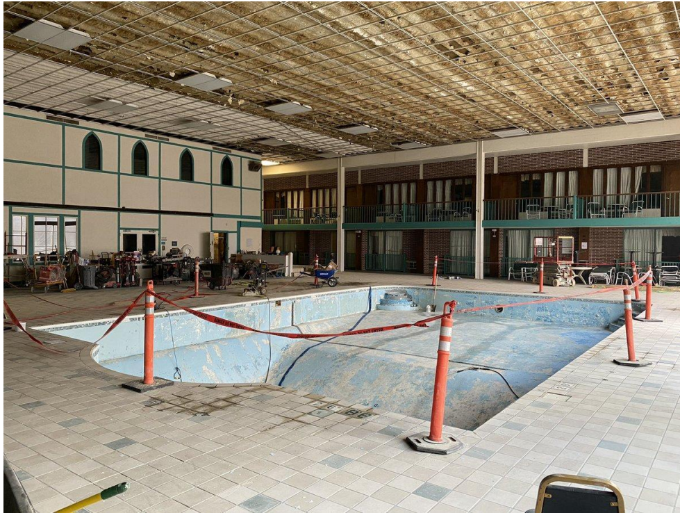
Photo 8-136: Rehabilitation of the pool area, December 2020, looking southwest
