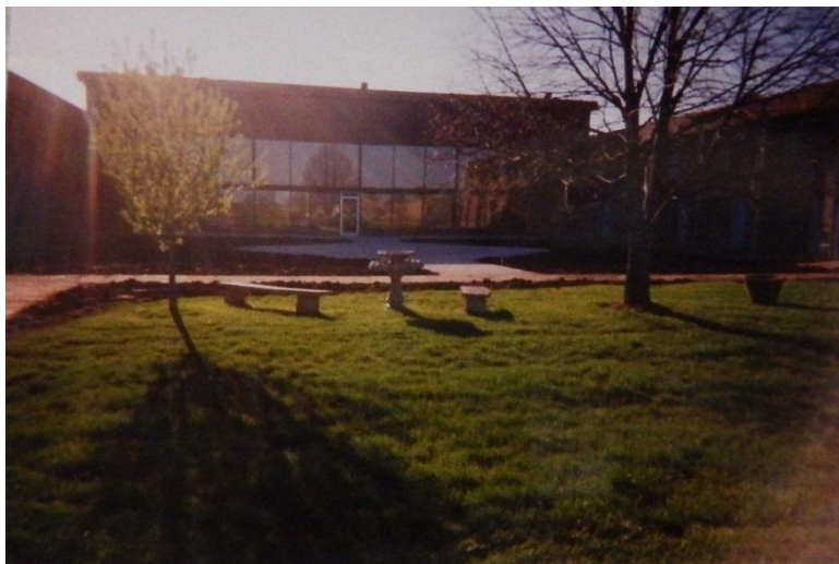
Figure 8-116: Original east pool/court windows, looking northwest
