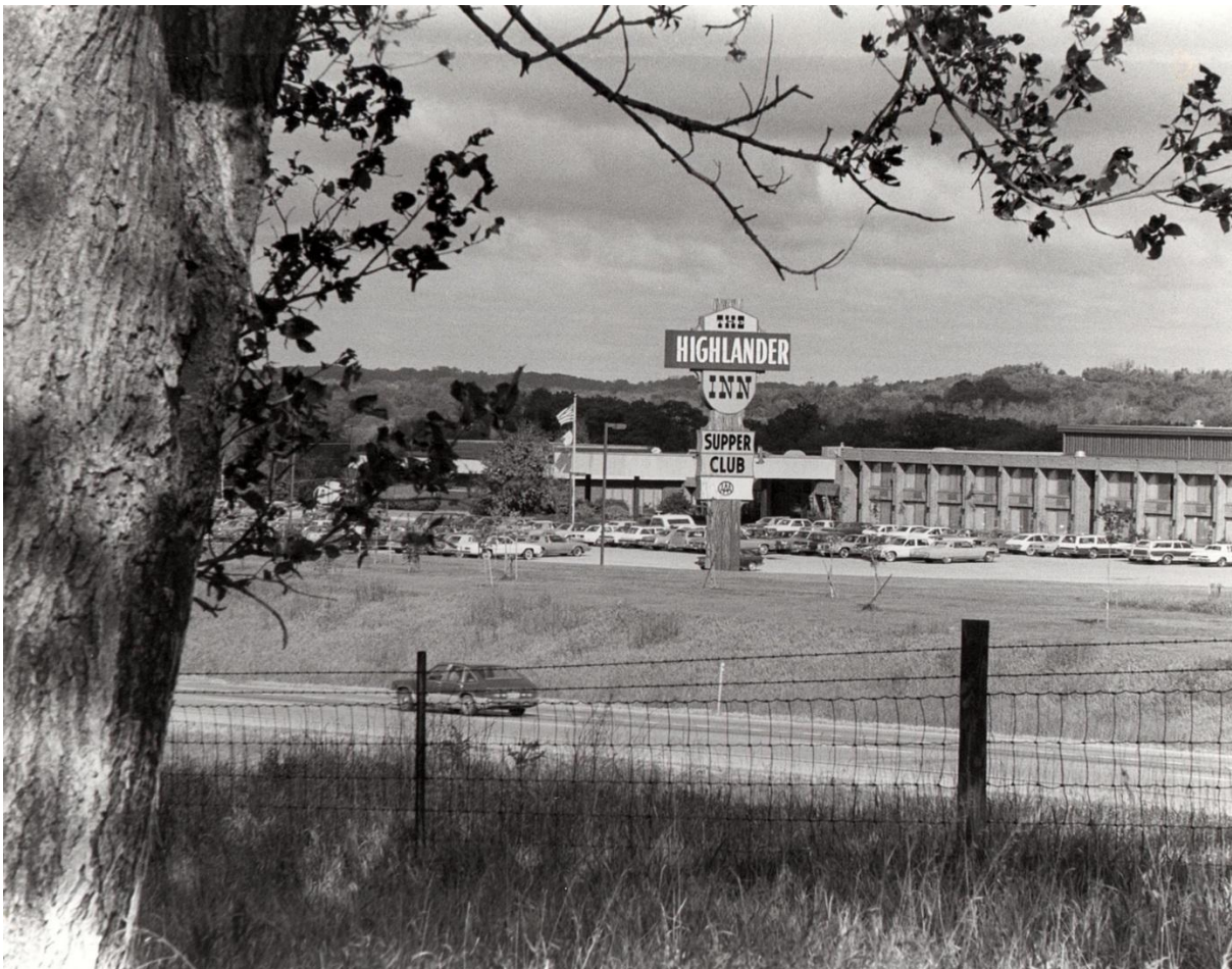
Figure 8-101: Overview, looking northwest (helicopter in Figure 8-77 visible far left), ca.1975
