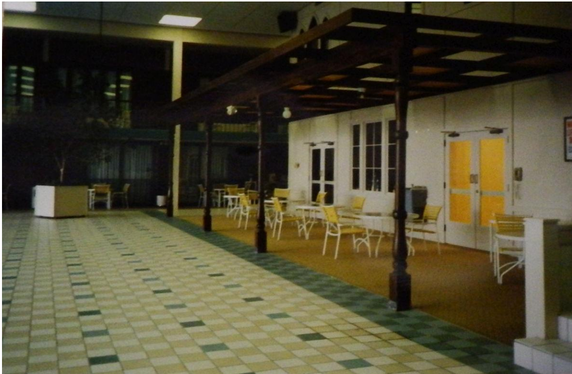
Figure 8-108: Tiled floor installed in the pool court, 1984, looking southwest (owner scrapbook)
