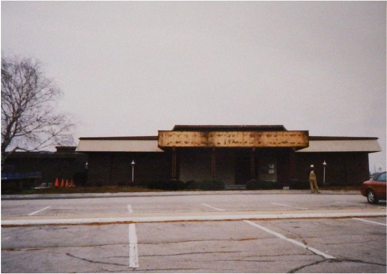
Figure 8-109: Demolition of west inn entrance, 1996, looking east (owner scrapbook) 30
