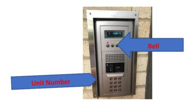
The Intercom handset in your Unit will ring. Pick up the receiver and you will be able to talk with the person outside, press the KEY button to unlock the door or Gate.
